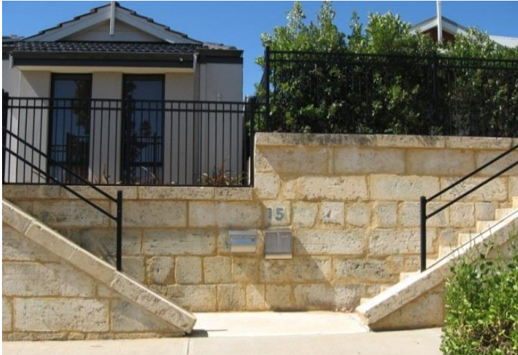
Figure 5: Stairways at Front of Properties
