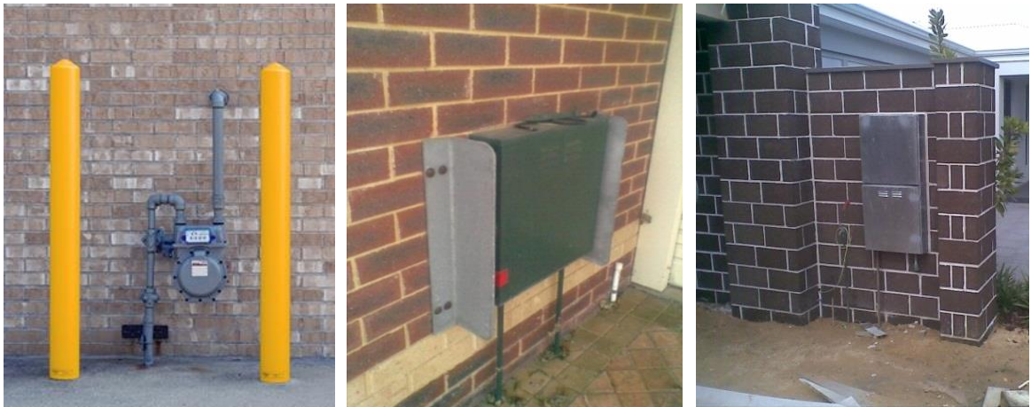
Figure 46: Gas Meter Box Protection (Examples)
