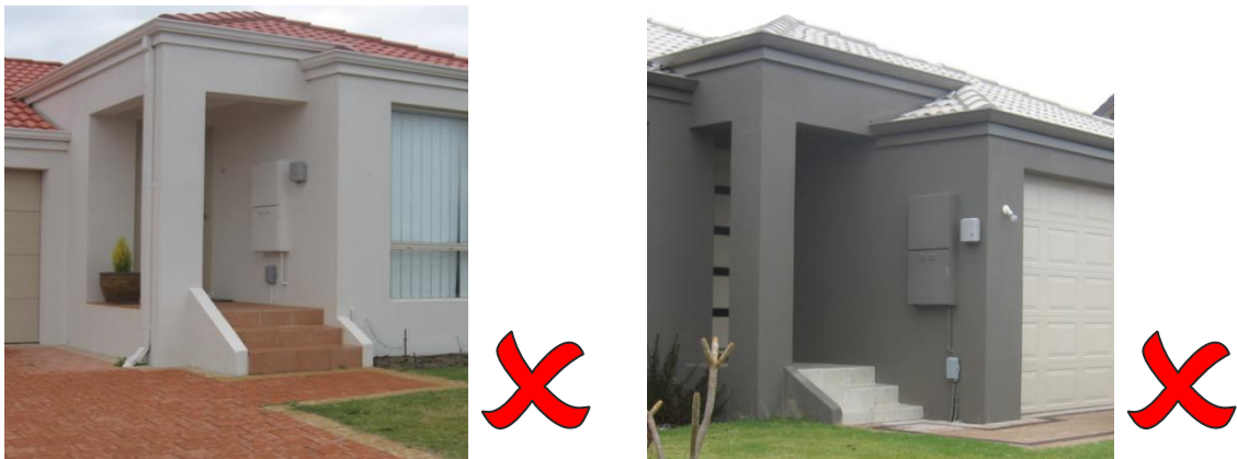
Figure 23: Gas Meter Box Installed Above Flight of Stairs (Unacceptable Positions)
